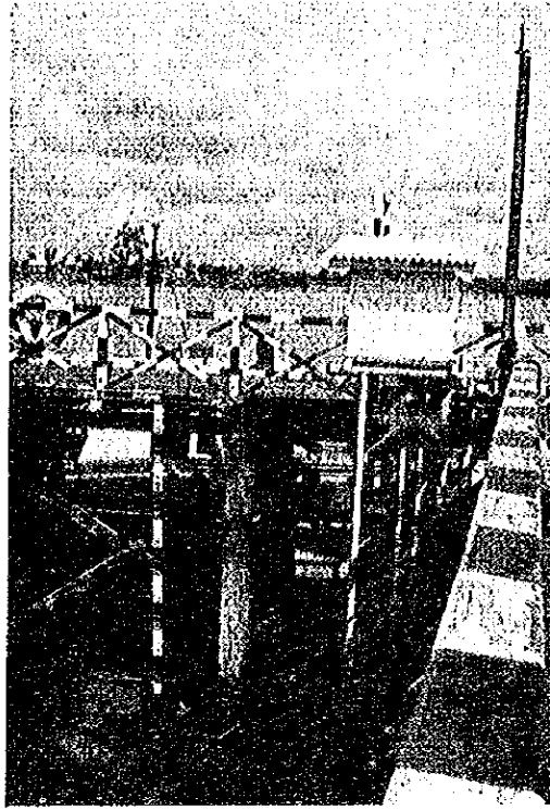
WATER GAUGE INSTALLED AT THE PENDING JETTY
