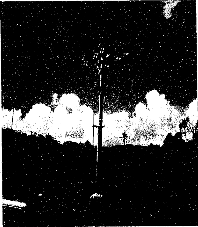
Concrete Pole and Distribution Lines installed in 1990 (South Area of Island)
