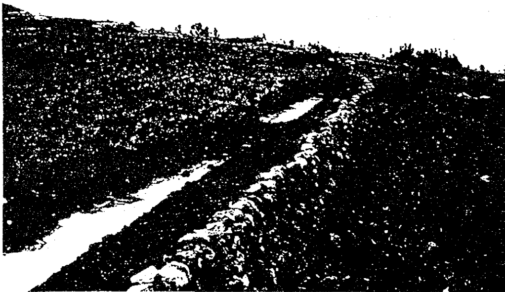
Contour bunds in Ethiopia, with ties in the basin and stone reinforcement of the bank (H. Hurni)
