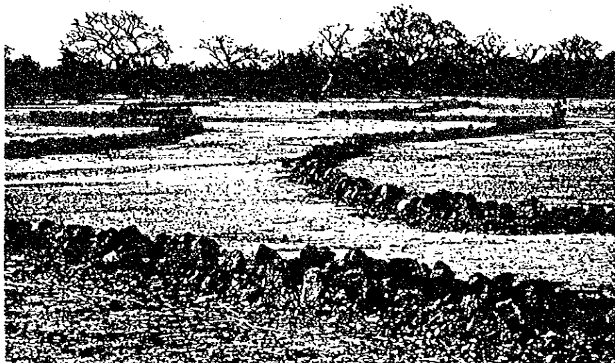
Stone lines set out on the contour near Onahigoua, Burkina Faso (OXFAM)
