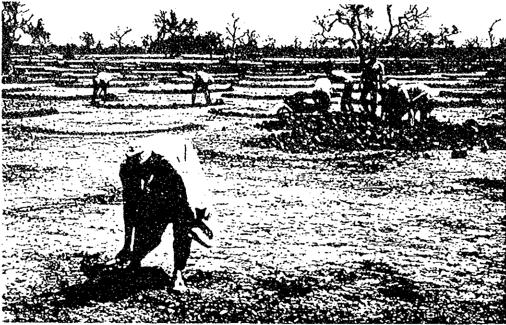
Marking out semi-circular hoops called 'diguettes' with a shallow excavation, Burkina Faso (OXFAM)
