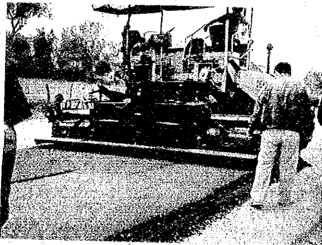
Base Course Material being placed by "Finisher".
