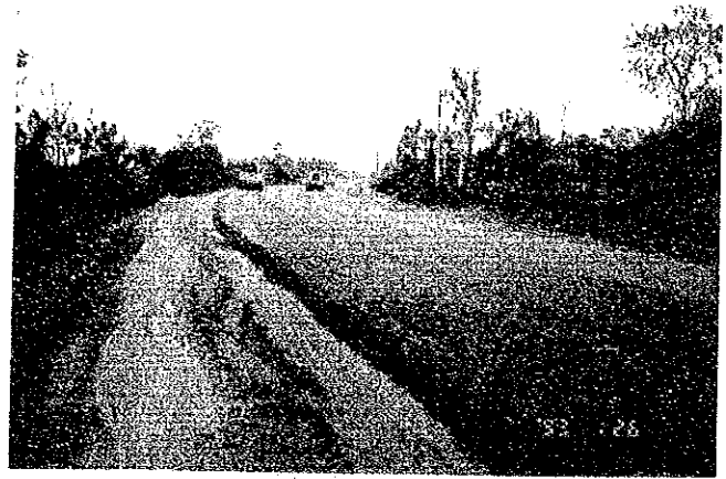
Base Course Work National Road 13S: aggregates be mixed with sand, lateritic solid (solid sandy soil with gravel) excavated at the borrow pits.
