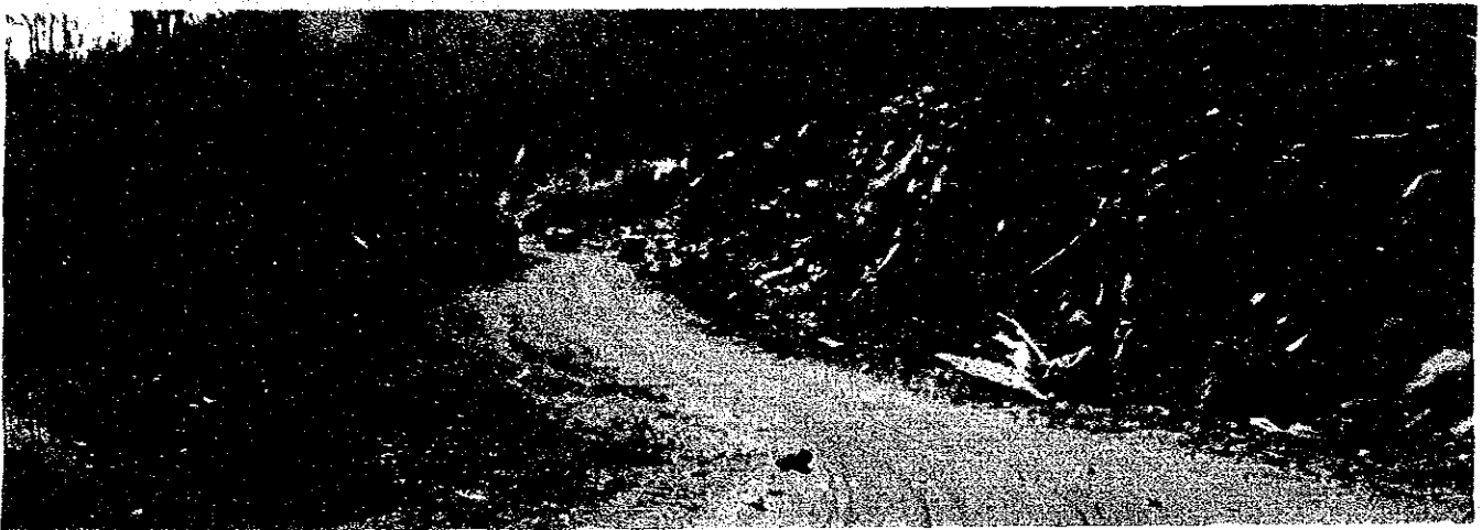
Rocky terrain, further excavation by blasting will be required. (Sta. 34 Km)
