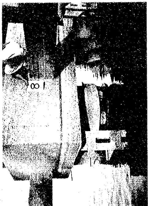
Photo 5-6 Octagonal concrete piles, concrete cells slipped down and horizontal beams which were constructed in 1960 as original structure. Concrete footing and steel batter piles were constructed additionally in 1983. Bent 8, Row A, of Berth No. 5.
