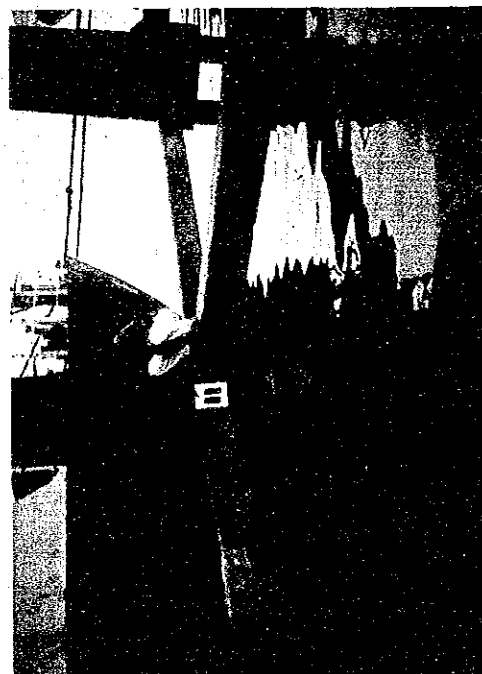
Photo 5-2 Concrete column and broken horizontal beam at Level 3, Bent 11, Row A, of Berth No. 4.
