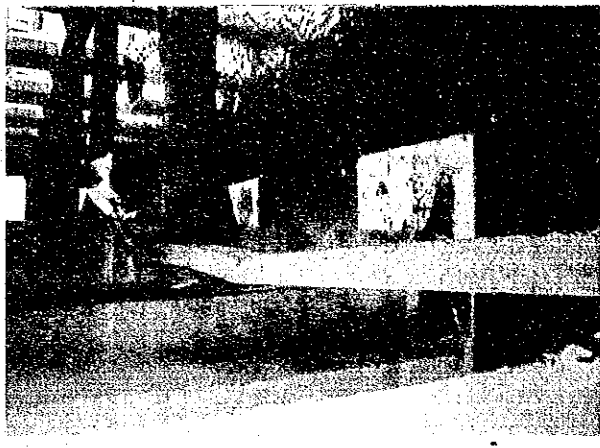
Photo 4-4 Exposed steel re-bars on the bottom surface of the top slab at Bent 8-9, Row A-B Photo taken on Dec.13 1992
