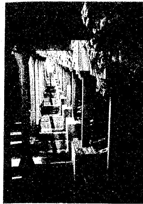
Photo 5-5 Horizontal beams, columns, footings and sediment at Berth No. 5.
