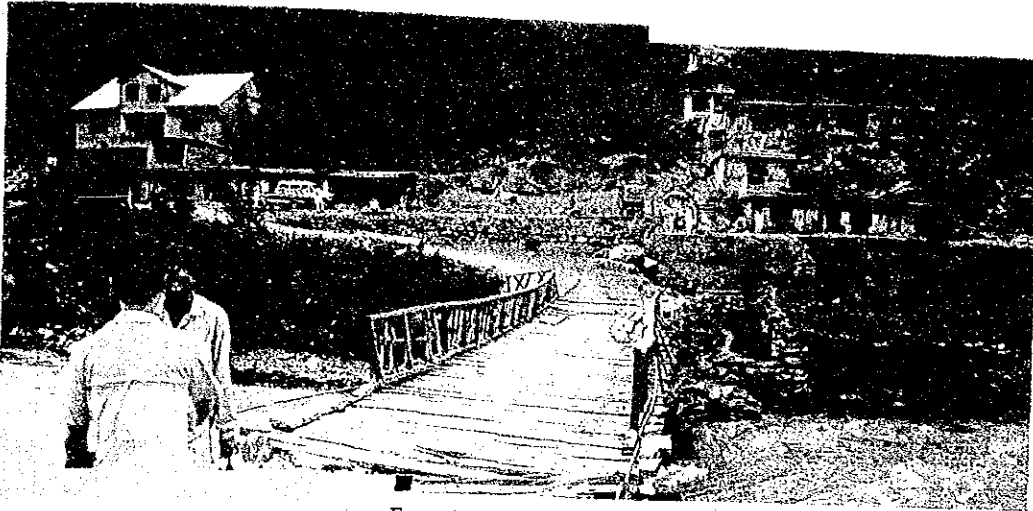
Front view of the existing Kaidon Bridge
