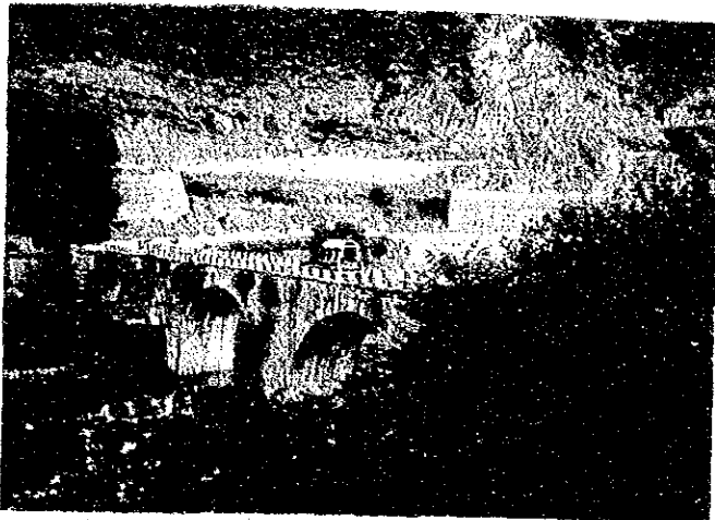
Downstream side view of the existing Jabrai Bridge
