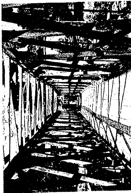
Condition of Floor deck (Wooden members are decayed seriously.)
