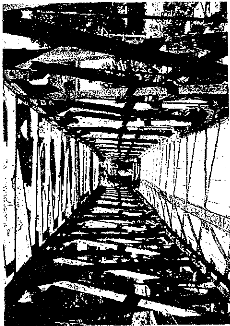
Condition of Floor deck (Wooden members are decayed seriously.)
