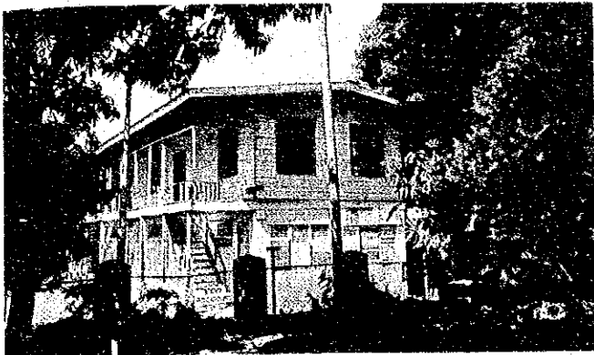
E-11 SAN JUAN SOUTH ELEMENTARY SCHOOL
