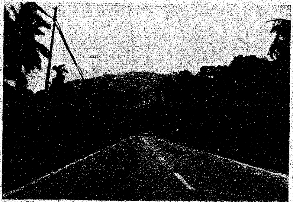
FEDERAL ROUTE NO 3 BETWEEN KOTA BAHRU AND KUALA TERENGGANU
