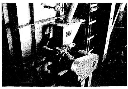
Limestone Feeder (Screw Feeder)
