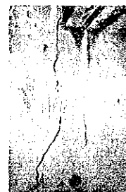
Vertical Crack on Wall
