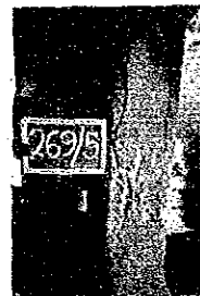
Longitudinal Cracks on Pier Column
