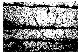
Flaking and Rebar Exposure on Deck Soffit
