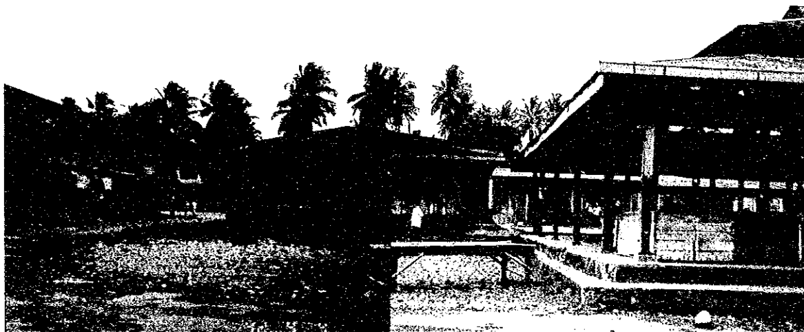
INSIDE PUBLIC MARKET SITE (REPAIR THE CENTER AND THE RIGHT SIDE RIDGE)
