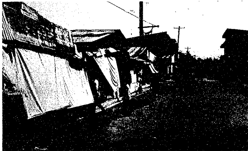
PUBLIC MARKET BARRACK GROUND (REPAIRING PART)
