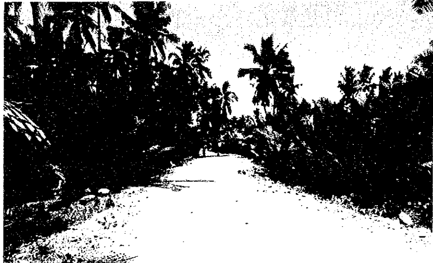
SLAUGHTER HOUSE NEW SITE'S FRONT ROAD
