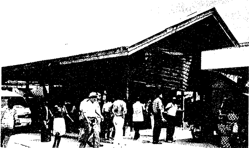
A PART OF REPAIR BUILDING
