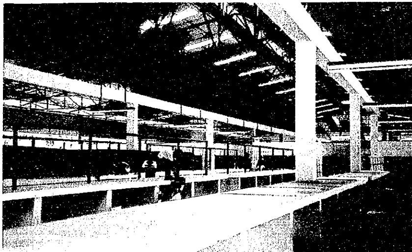
INSIDE EXISTING SLAUGHTER HOUSE INSIDE
