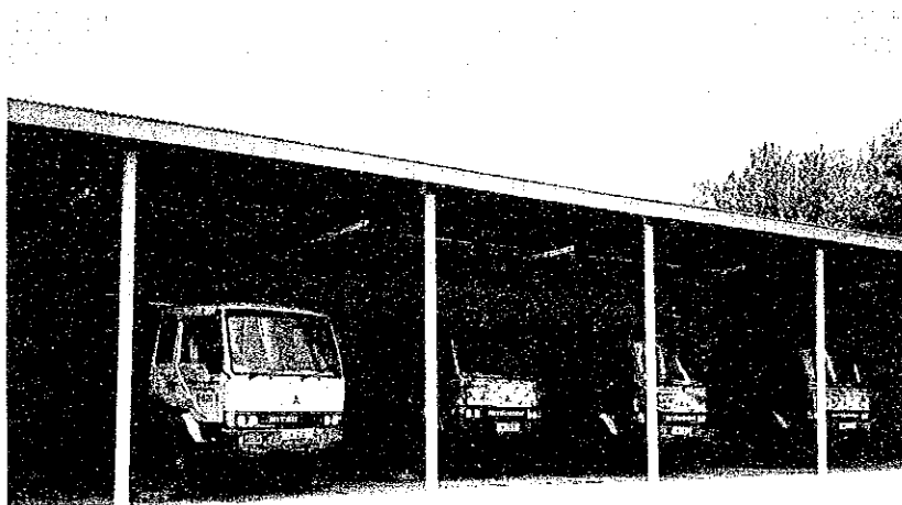
MOWTC Fort Portal Area Office Workshop and depot/
