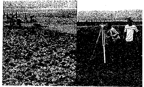
Farm levelling work
