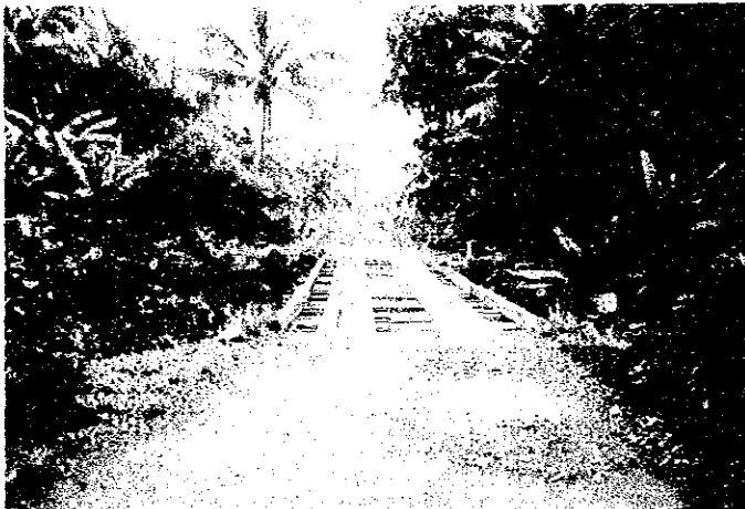
No. 8 Bridge No. ; 05.04.03 Bridge Name ; Pinaglagaan Bridge
