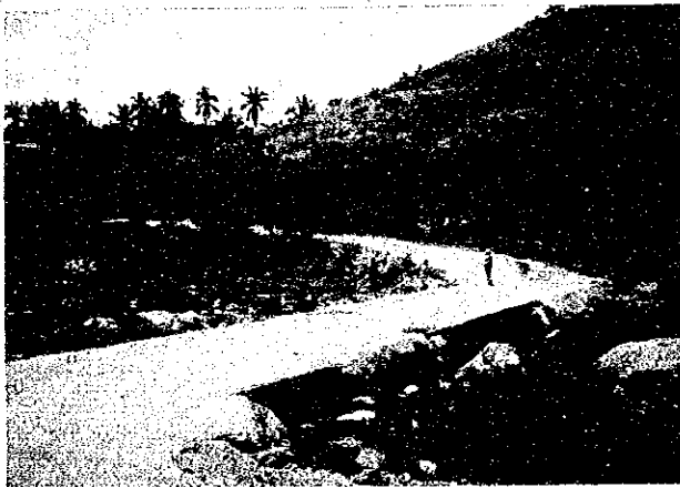
No. 3 Bridge No. ; 05.06.04 Bridge Name ; Lanang Bridge
