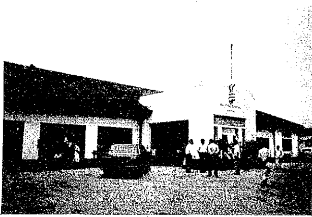
Provincial Hospital, Kalutara (general hospital)
