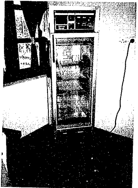
New blood refrigerator: currently not used because no surgical operation is performed.
