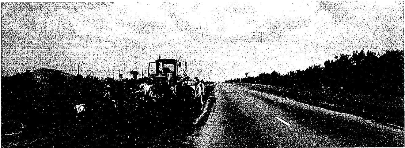
National road near Mojo. The surface is smooth. Shoulder is under improvement.
