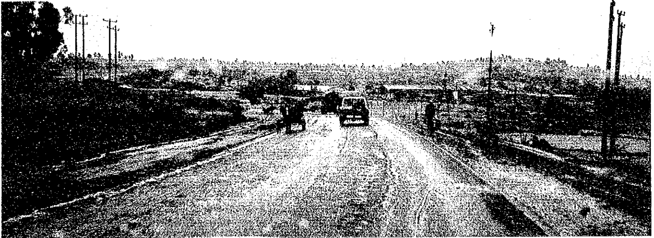
National road in the suburbs of Addis Ababa. Irregular surfaces after the partial repair will need additional repair.
