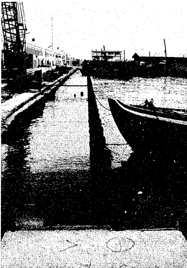
Photo-14 SHEET PILING SEAWALLS (Sep. 1991)
