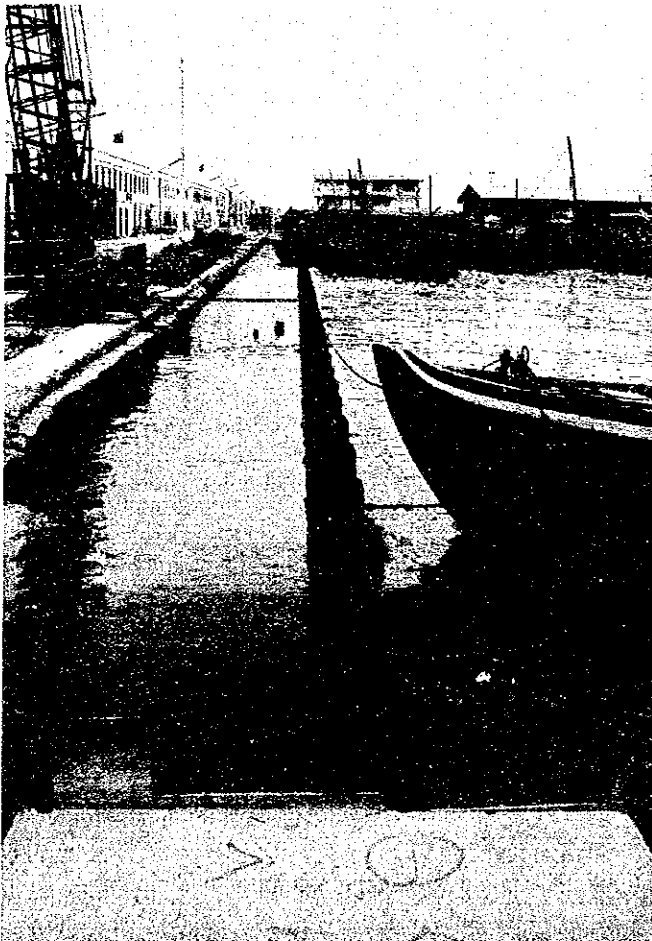
Photo-14 SHEET PILING SEAWALLS (Sep. 1991)
