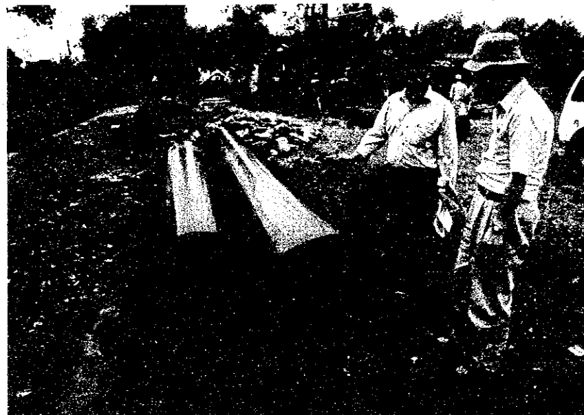
Drive casing pipe damaged by Boulder during cased hole drilling
