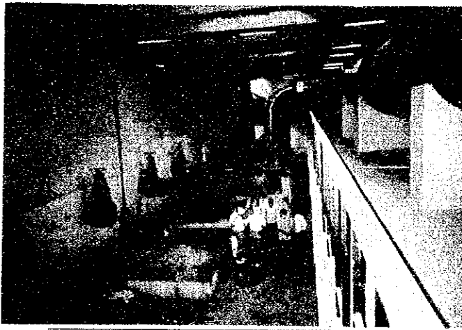
Inside of pumping station for 6th October Waterworks (intake pump room)
