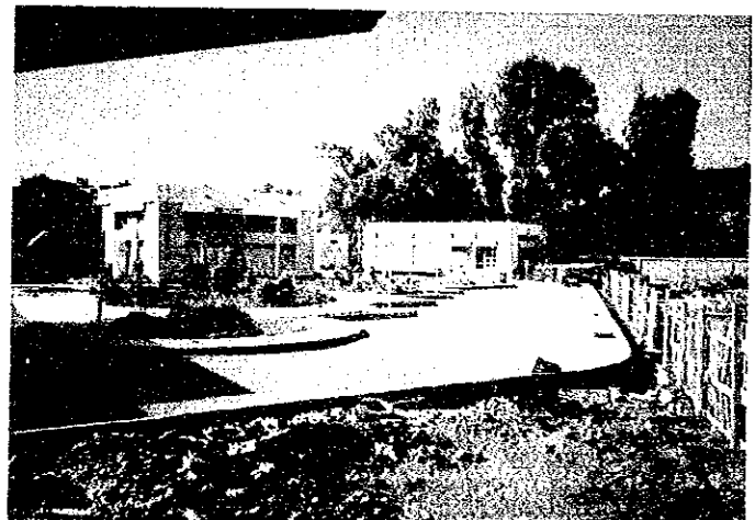
Sewer Transfer Pump Station No. 5 (A) building (left) and sub-station/emergency power generation facility (right). The wooden fence on the right marks the boundary between the No. 5 (A) and No. 5 (B) stations
