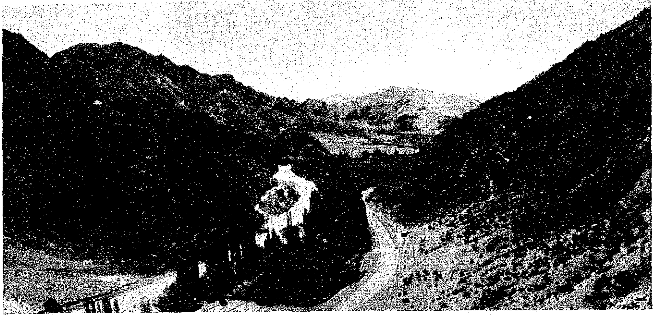
Olur Dam Site
