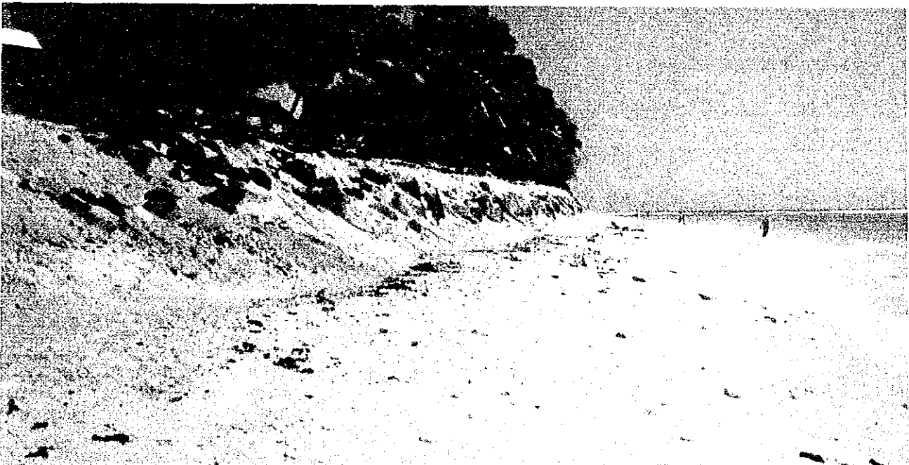
Edge Water Hotel being built too close to the beach, urgent sea wall was constructed, Tokorau District
