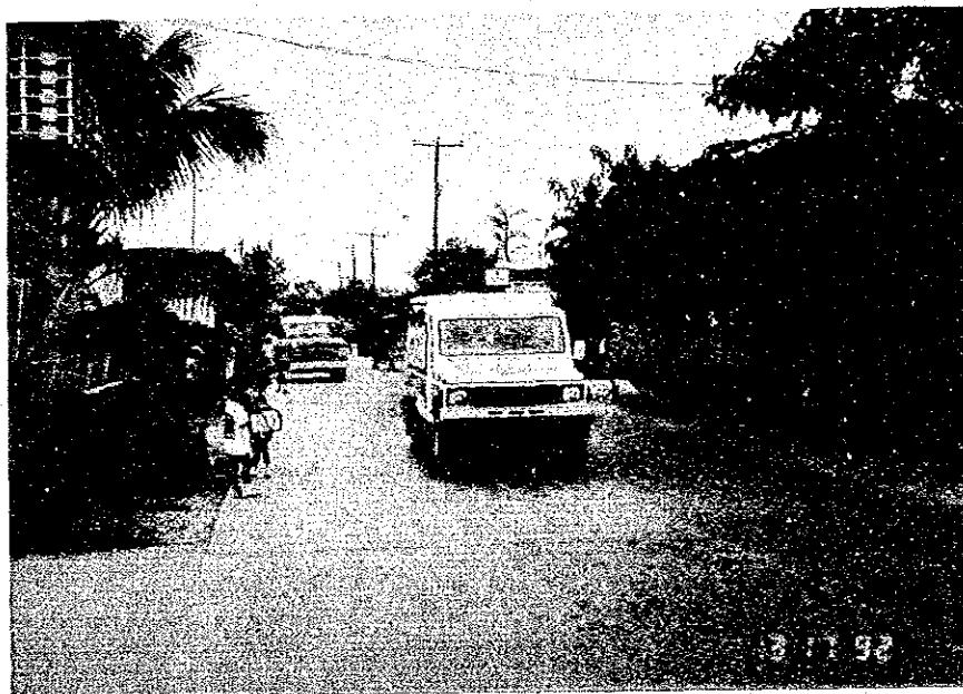
Photo 10-8 Existing Road Condition Connected to Ro/Ro Terminal (Bacolod)
