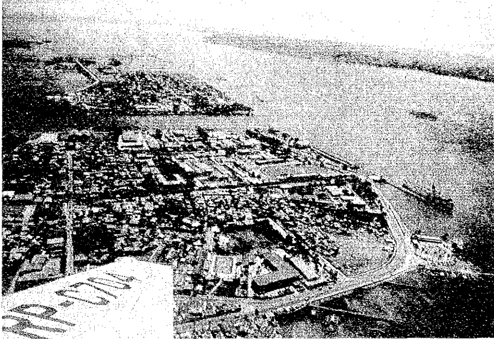
Photo 5-3 Port of Iloilo (Old Foreign Pier) Source: JICA Study Team
