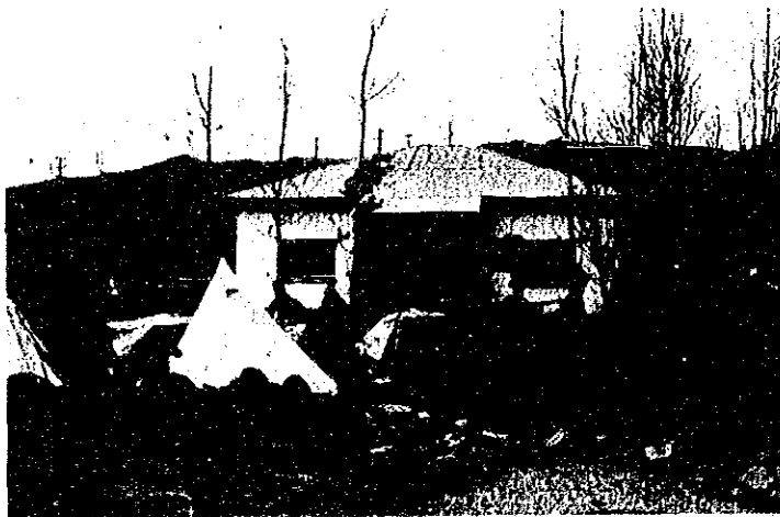
Fig. 28 Slightly Damaged Local Dwelling in Muradiye.
