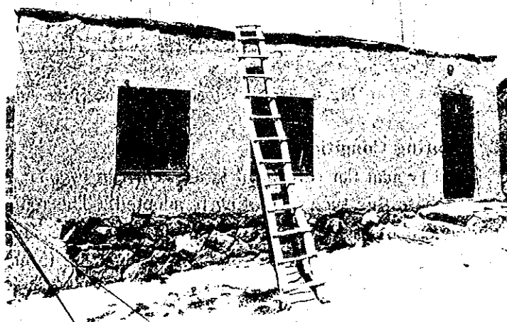
Fig. 3 Adobe House from Muradiye.
