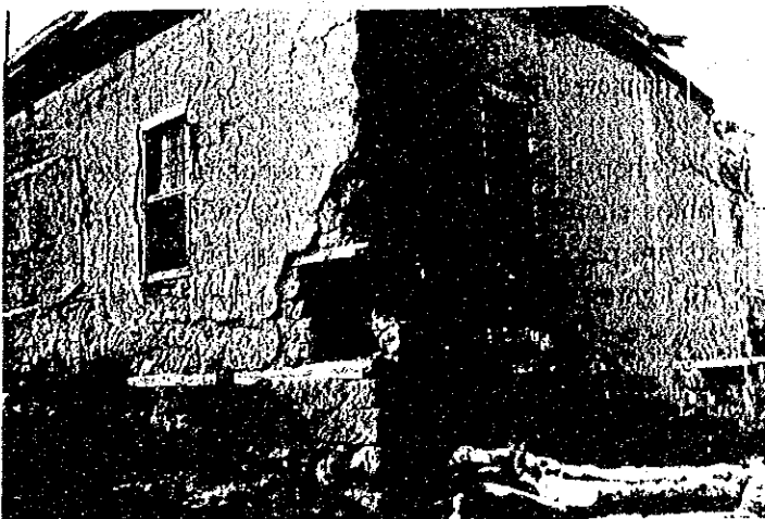
Fig. 12 Lintels to Prevent Corner Damage.
