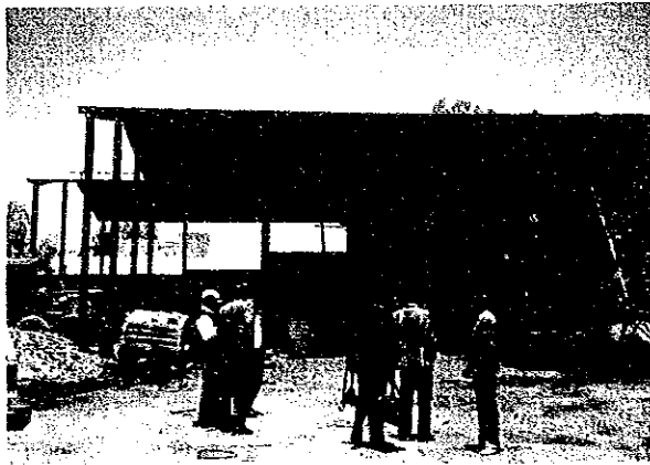
Repairing Shop at Existing Workshop in Sana'a
