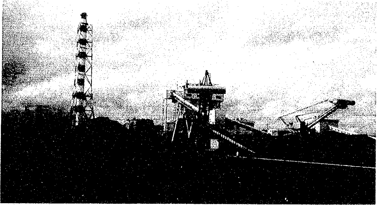
Batangas Coal-fired Thermal Power Plant
