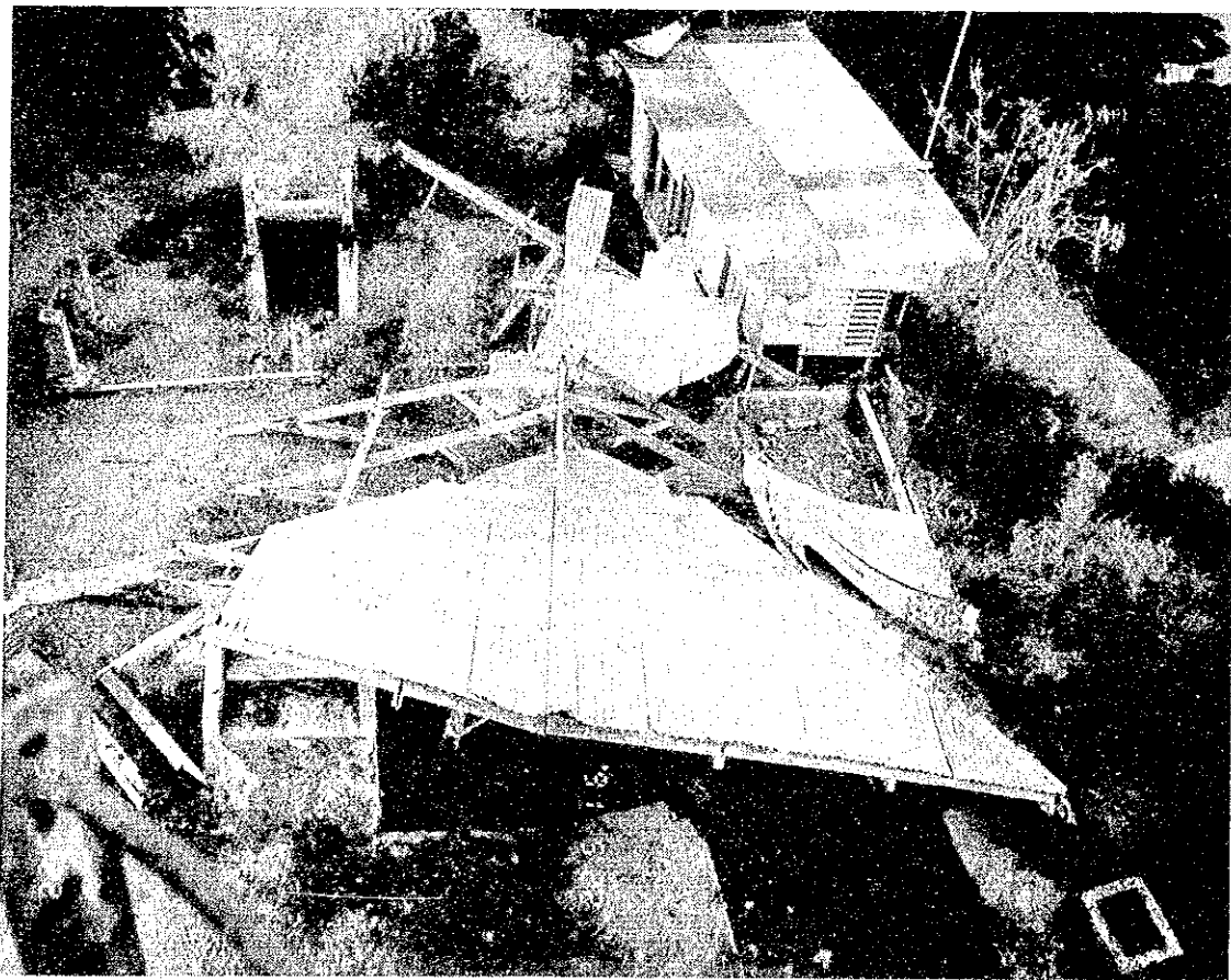
Picture 19-2 Broken associated building by typhoon
