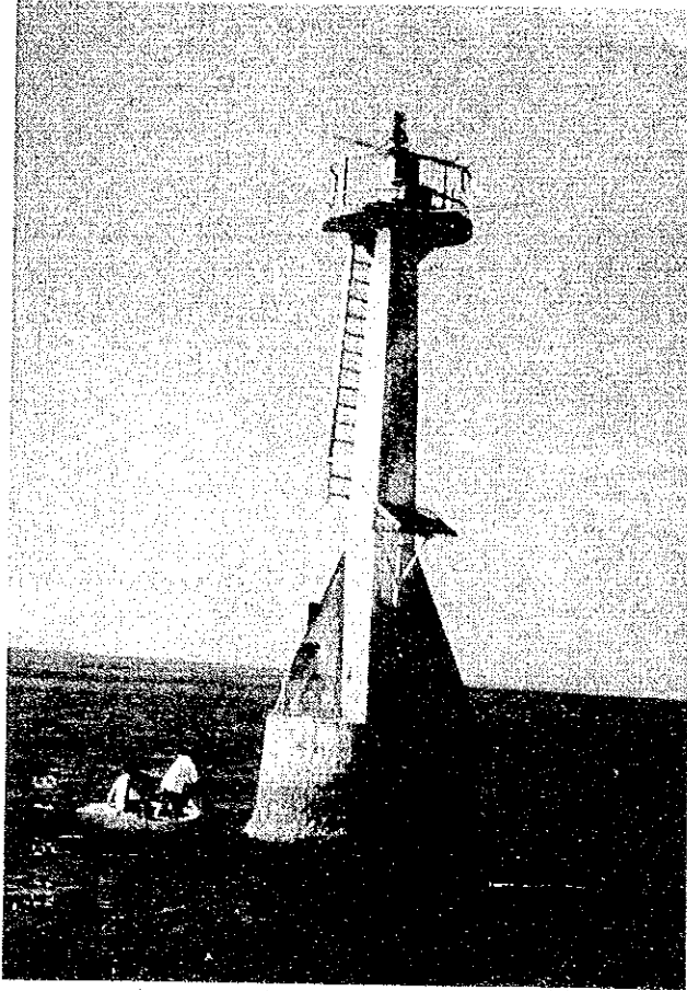
Picture 11-1 Inclined Structure
