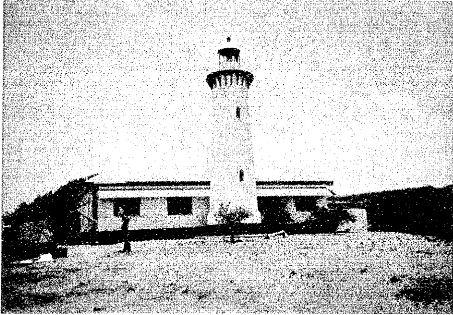
Picture 1-1 : Overview of Cape Santiago LH
