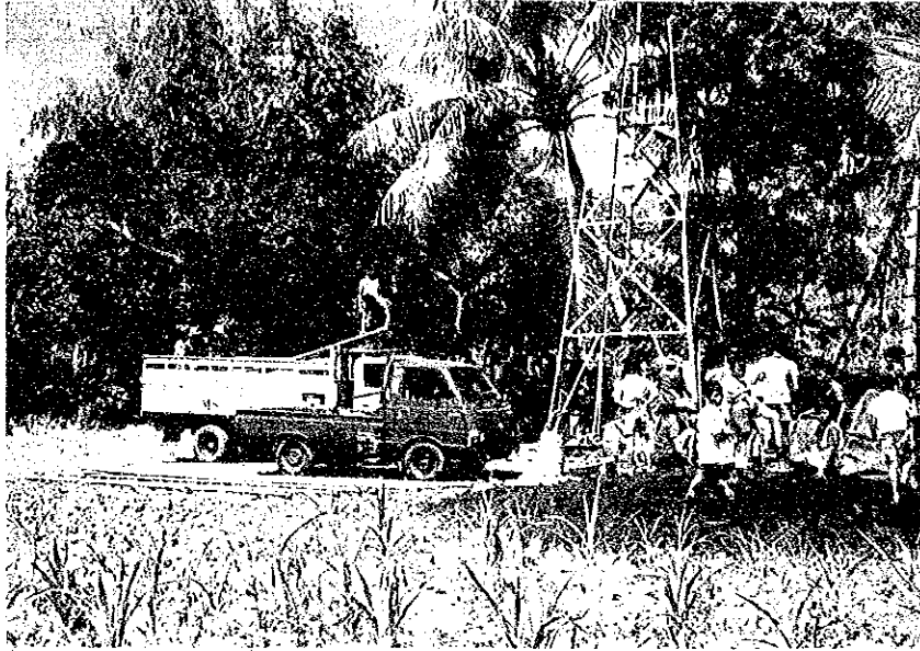
Drill rig mobilization, Banyuanyar August, 1991
