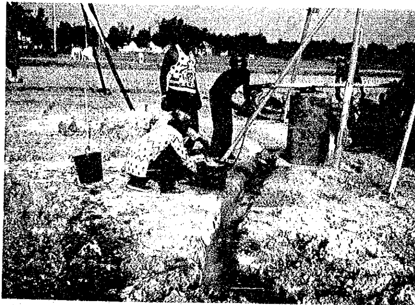
Trial pumping of test well at Jepon August, 1991
