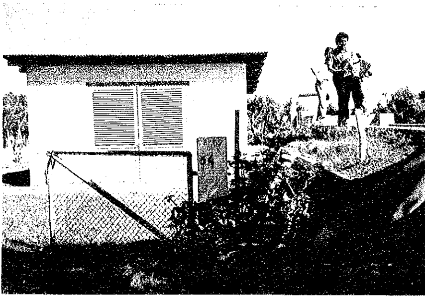
Pump Station of P2AT SP-67 Well in Desa Suwalan
