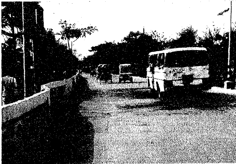
Concrete Flood Wall of DND project Zone
