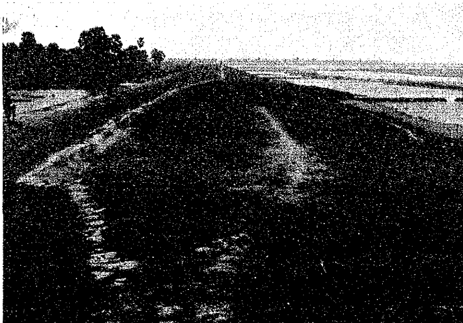
Slope Failure Section of Embankment Nearby National Zoo
