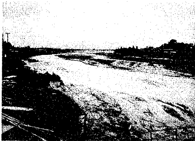
Abacan Bridge: Scouring upstream
