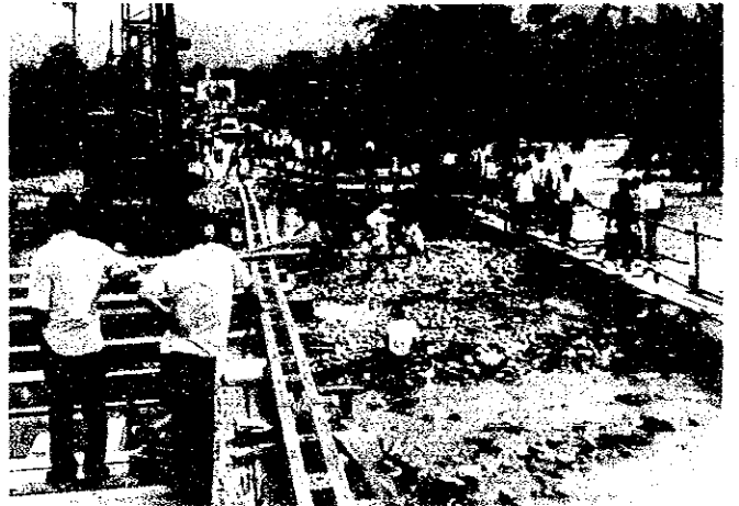
Construction of Tentative Bridge
