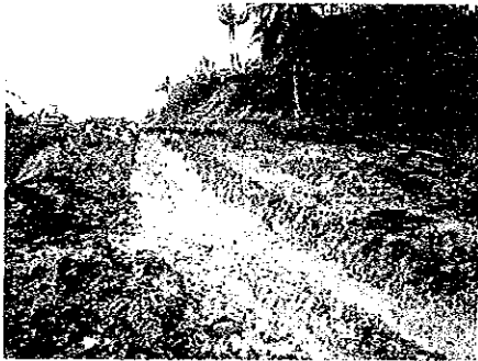
7. Flooded/Muddy Road Surface (FM-Rd) Spot L - 23 (Leyte)
