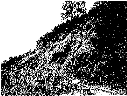
1. Cut Slope Failure (C-F) Spot Bt - 43 (Benguet)
