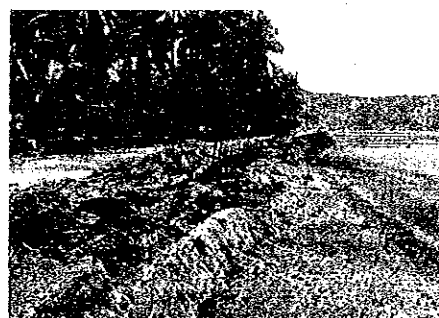
16. Seawall Damage (SW - D) Spot Bs - 51 (Balangas)
