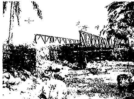
12. Temporary Bridge Approach Washout (TBr - A) Spot L - 38 (Leyte)
