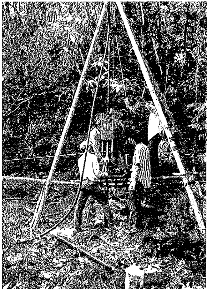
Drilling Work of Geological Investigation (KI-2)
