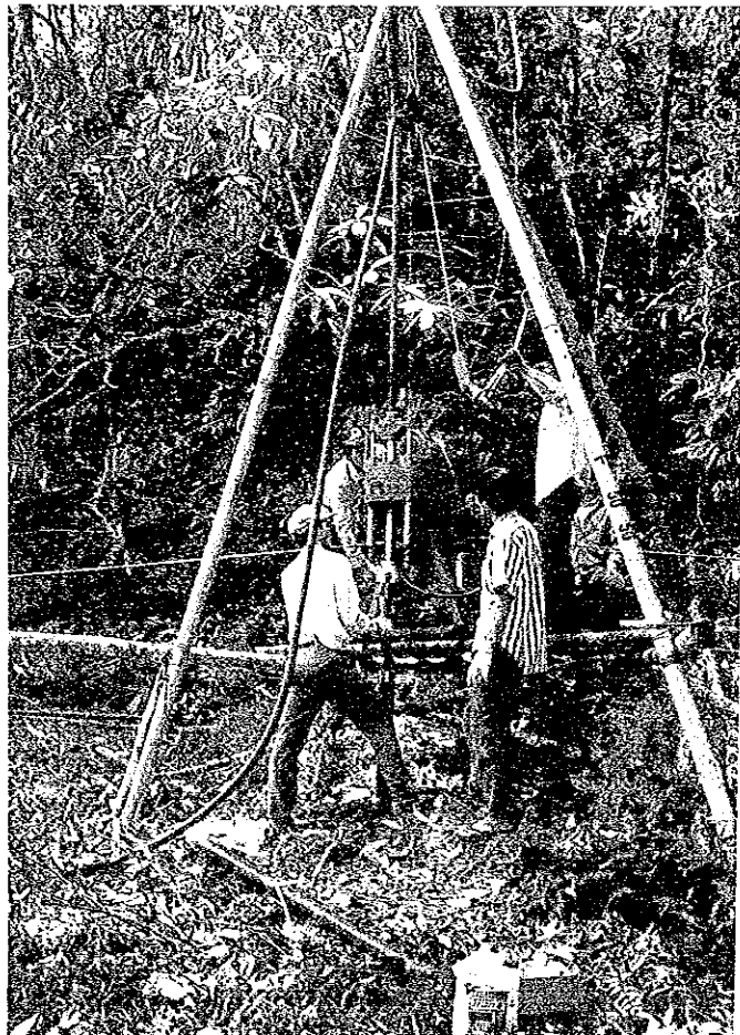
Drilling Work of Geological Investigation (KI-2)
