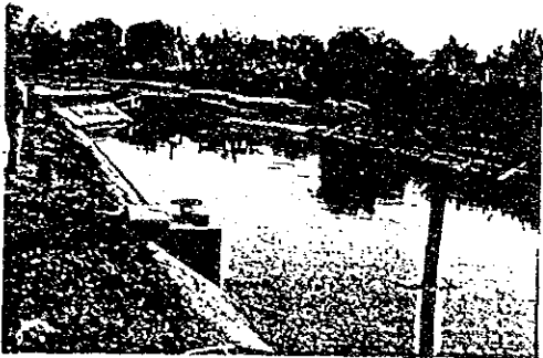
Photo-2 Constant head orifice offtake regulator
