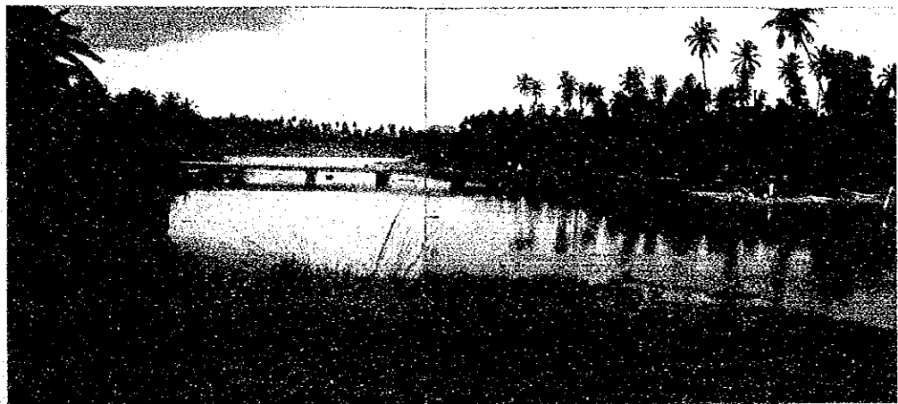
VIEW OF THE BRIDGE FROM DOWNSTREAM
