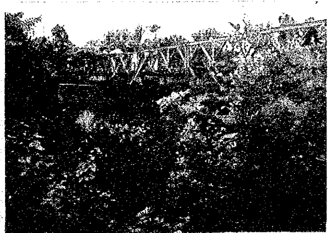
A VIEW FROM LEFT SIDE OF 1ST APPROACH
