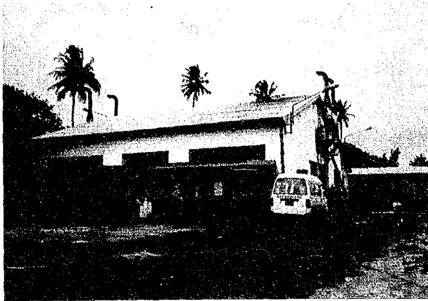
General View of UNELCO Luganville Power Station
