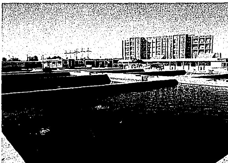
FMC experiment ponds (backside bldg. is the High Dam Lake Development Authority)
