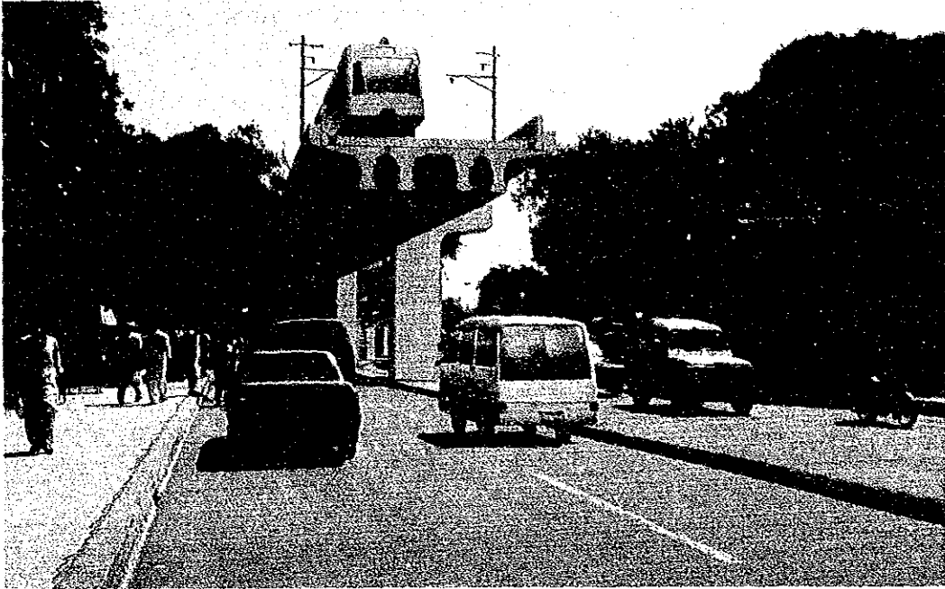
LRT ALONG THE MALL
