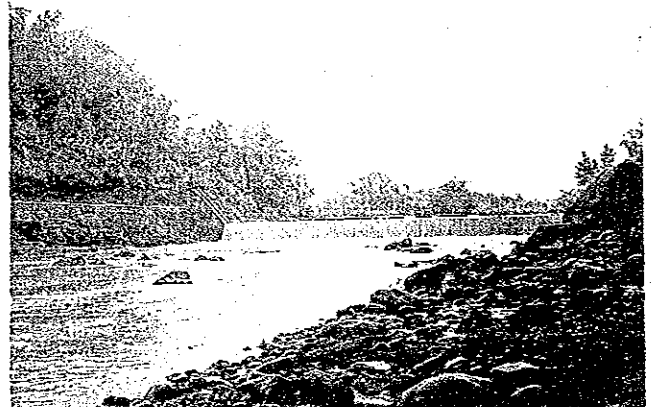
Check dam constructed in the upper reaches of Wonogiri dam
