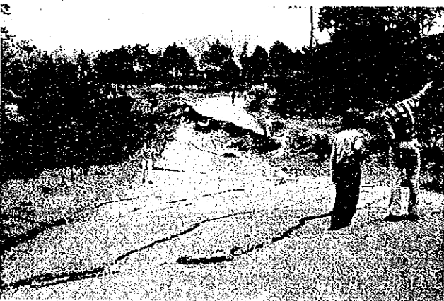
The landslide of Puncak, West Java occurred across the national road connected between Bandung and Jakarta. The old national road was destroyed due to the landslide and the new road was reconstructed at the upper side of the old one.
