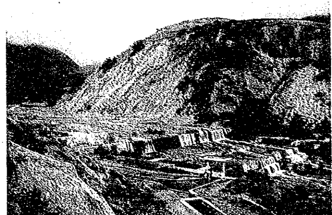
A check dam constructed on the foot of slope erosion in the Sombe river
